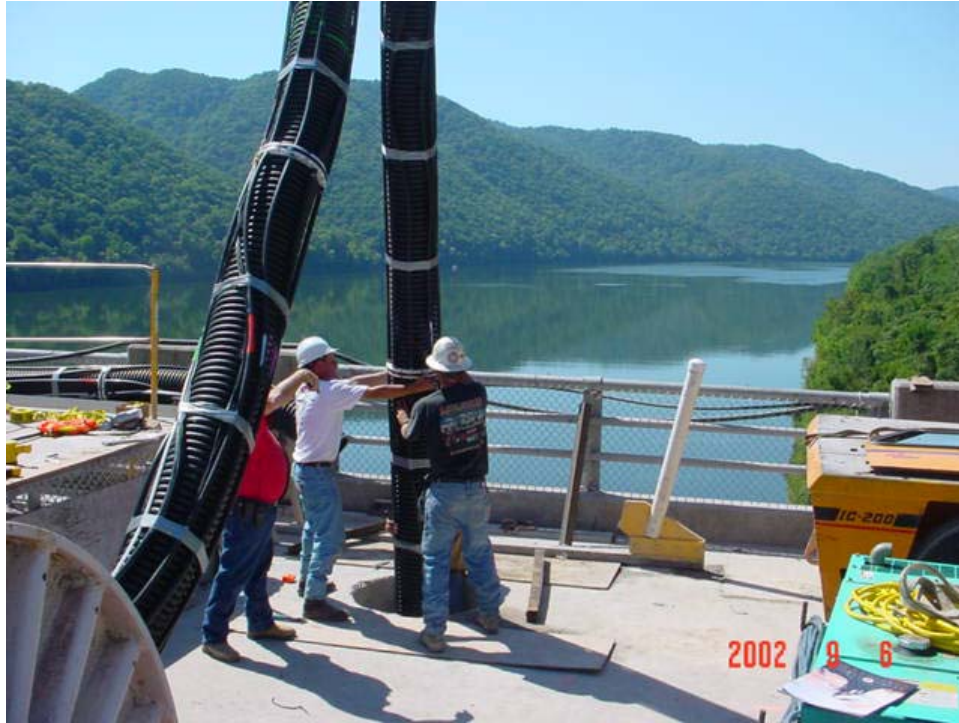
Figure 2. Fully Encapsulated Multi-Strand Tendon
